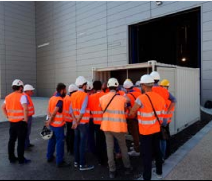
Container in front of the cable hall (left) Container operating area (right)
