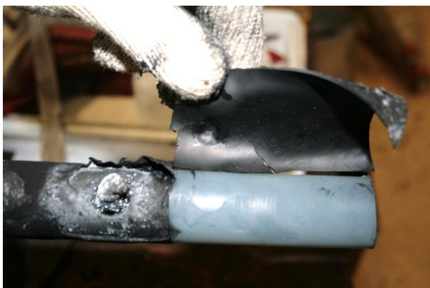
Water sign noted in insulation screen
