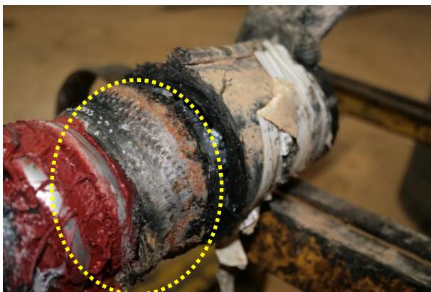
Fault point on L3 at Sumitomo
