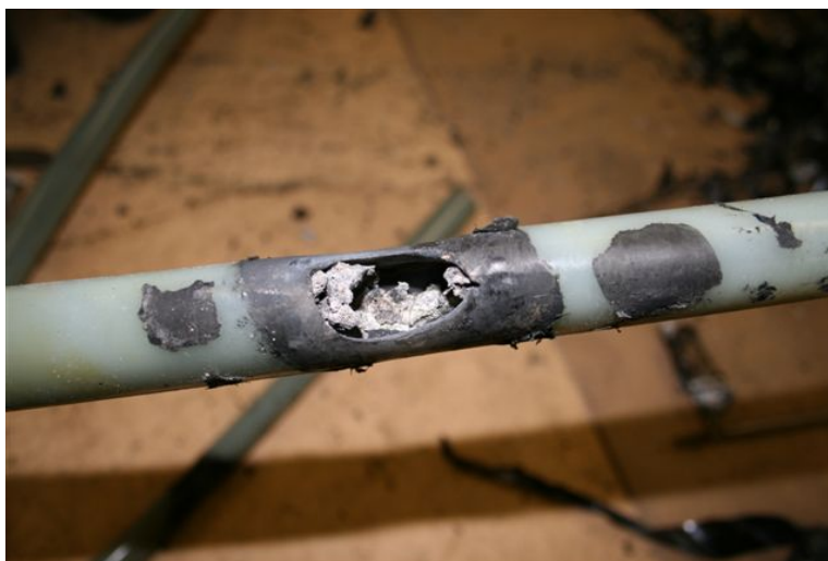
Cable body fault, L2 at 125m
