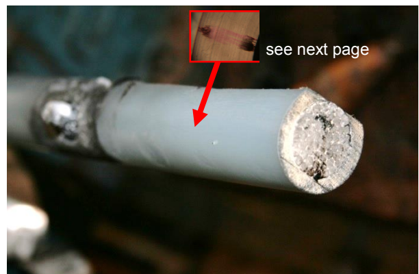
Suspected water tree developed near to fault point
