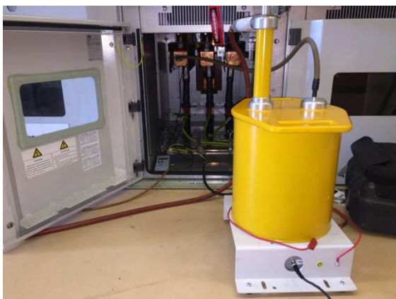
Figure 2: Combined VLF TD and PD diagnostic, field application
