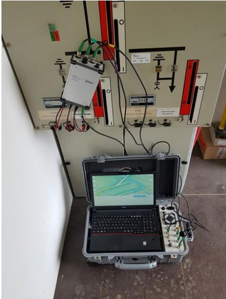
*Connect whilst energised, measure while energised: The new VDS-C can identify partial discharges on cables quickly and easily. (Image: Mitnetz Strom)*
