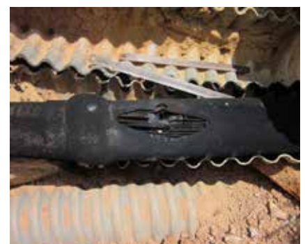
➤ Cable fault, 1-core 11 kV joint failure
