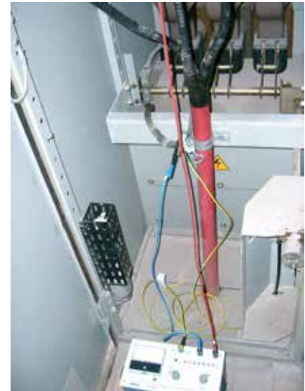
➤ galvanic connection of audio frequency generator TG
