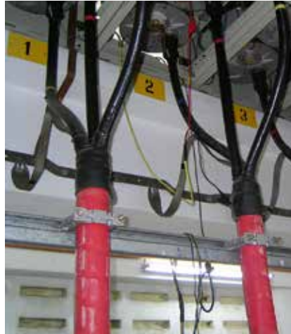
➤ accessible cable termination; calibration on full cable diameter
