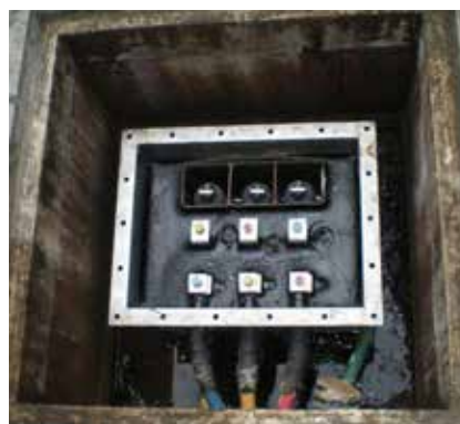
➤ Link box with open link connectors at 6814 m
