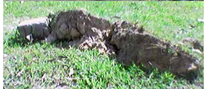
➤ exploded 132 kV joint after cable fault, 132 kV XLPE, explosion lifted soil above the faulty spot.
